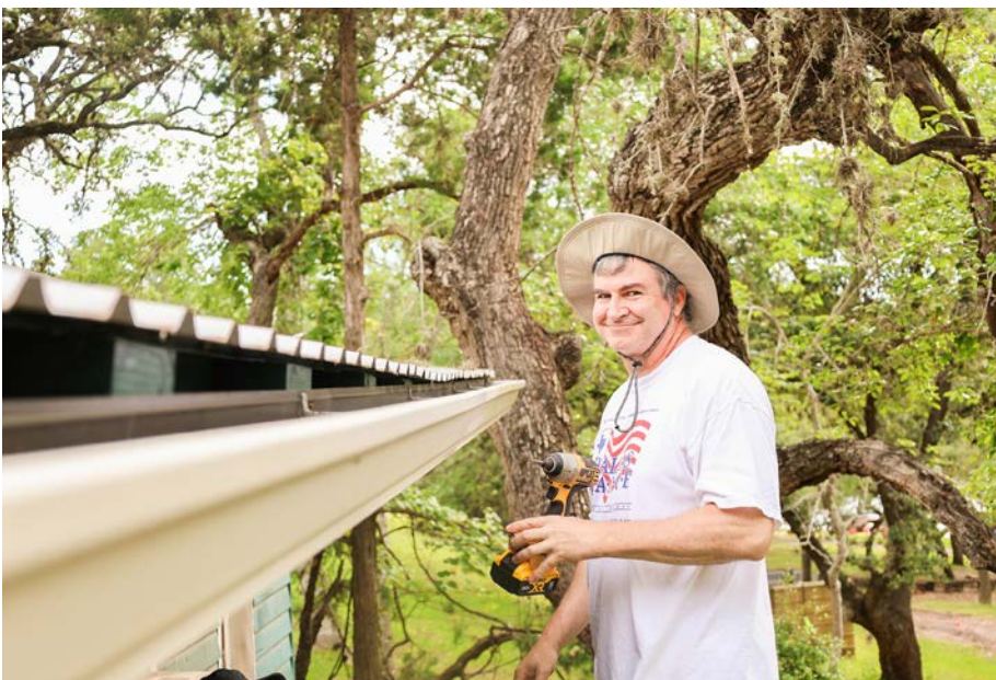
A volunteer helps with a gutter project at Camp Lone Star.
